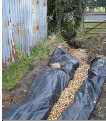
Land drain piped to ditch.
