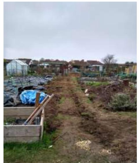
Row 26-27. Land drain installed and plot holders have started to back fill the trench.
